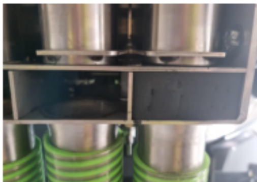
Foam block installed in gallery
